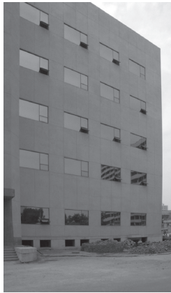
KUT Library Construction, 2004
